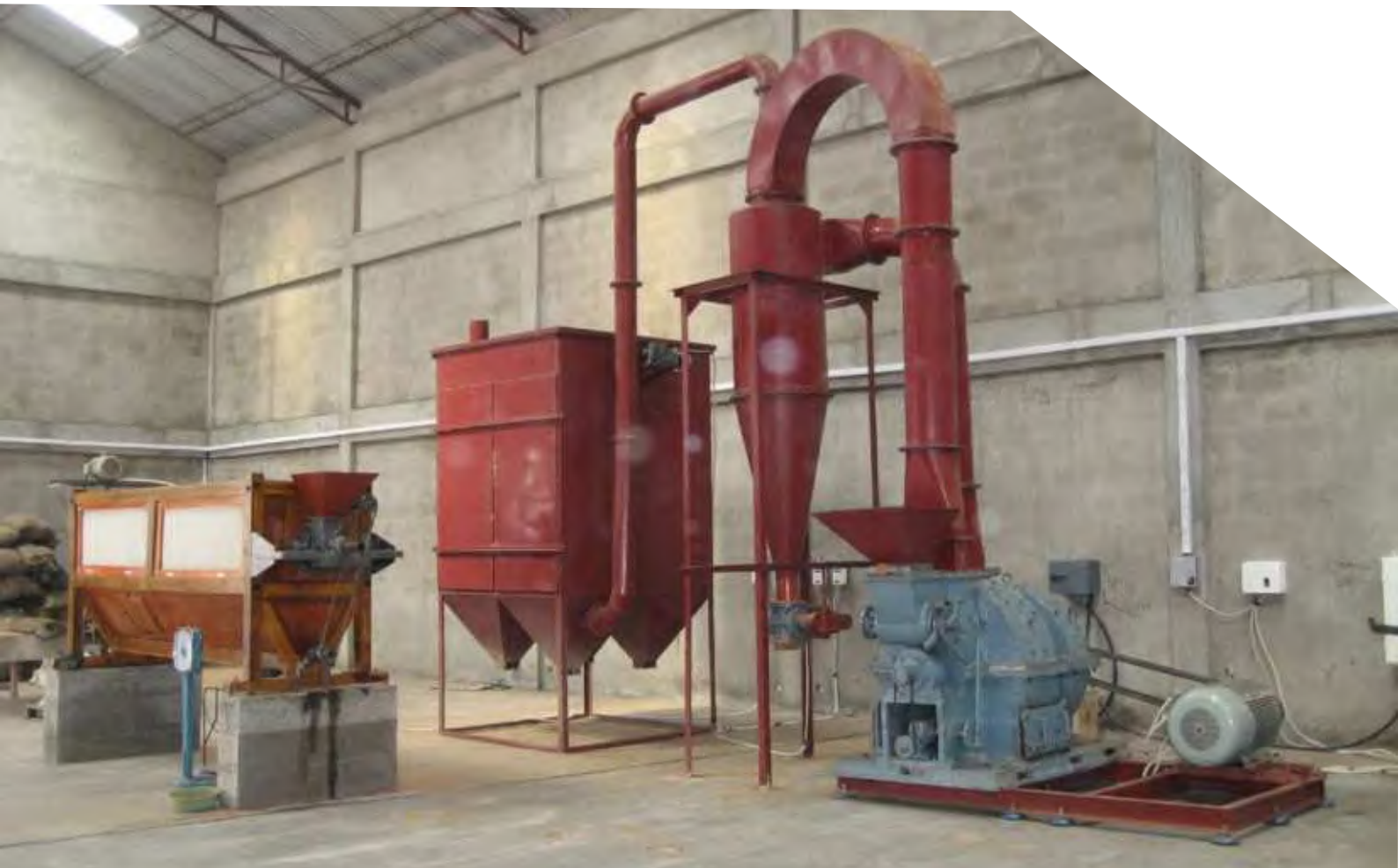
► Installation of DP IP-42 in Ghana, Africa
